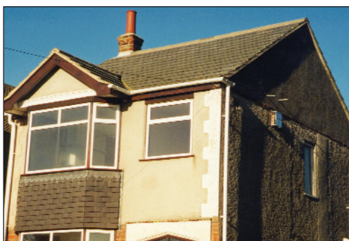
Closer view of main windows
